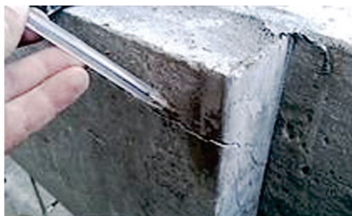
c) Grout rupture
