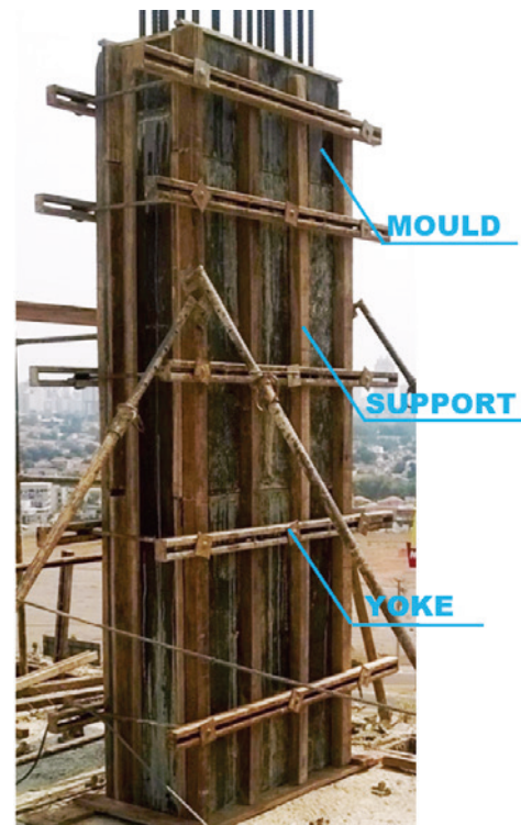
Figure 7 Constitutive elements of a column formwork
