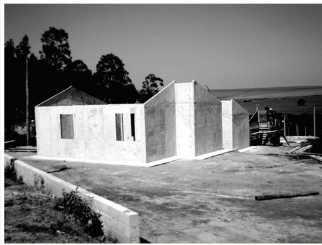
Figure 2 – Housing and walls constructed (10)
