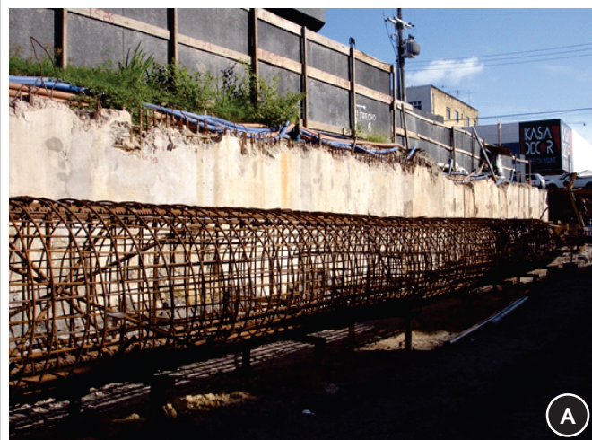
Figure 2 – Example of application of reinforced concrete circular cross section elements working as beams in a shallow tunnel (Maffei, (9)): (a) details of the reinforcement; (b) concluded beams
