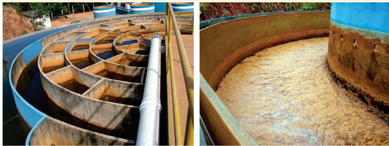
Figure 1 - Water treatment station in Santana do Paraíso-MG
