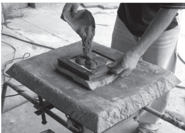
A Bearing pads casting
